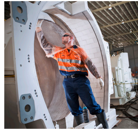
Applying WEAR MAX® to centrifuge housing
